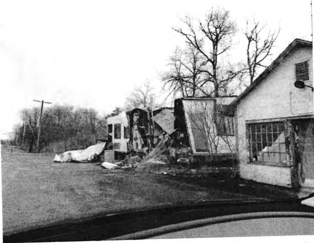
Attachments: views of multiple abandoned properties at the intersection of East Hill Road and State Route 52
