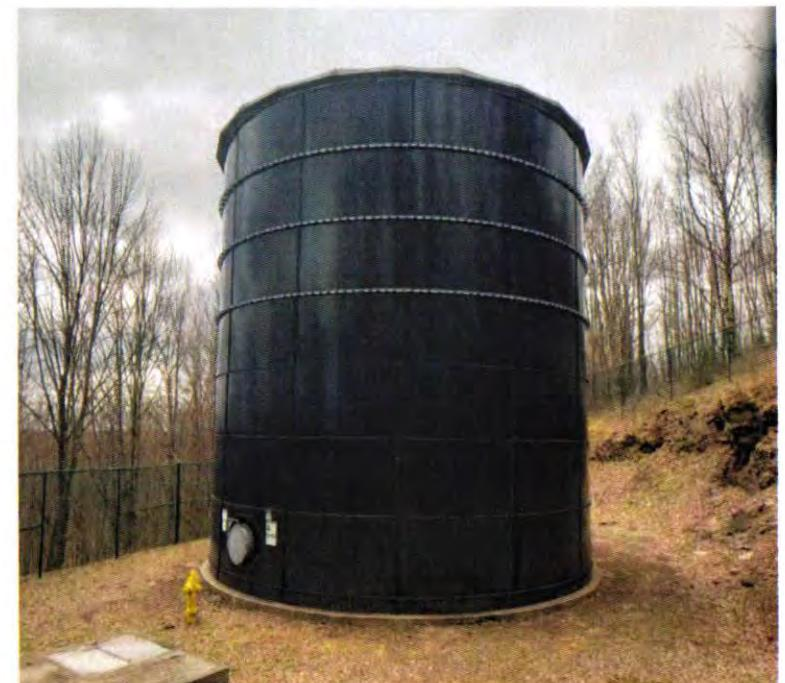
**NOTES:** 256,000 gallon capacity; bolted steel tank. Site improvements include: fencing.
