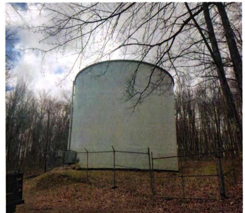
NOTES: 254,000 gallon capacity; welded steel tank. Includes: valve vault. Site improvements include: fencing.
