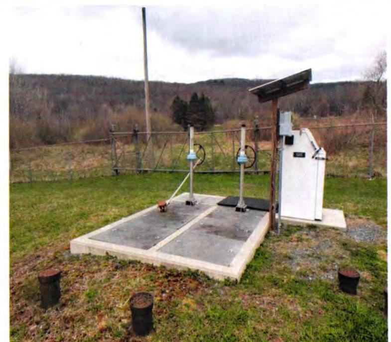
**NOTES:** Includes: parshall flume, flowmeter, valves, and sampler.
