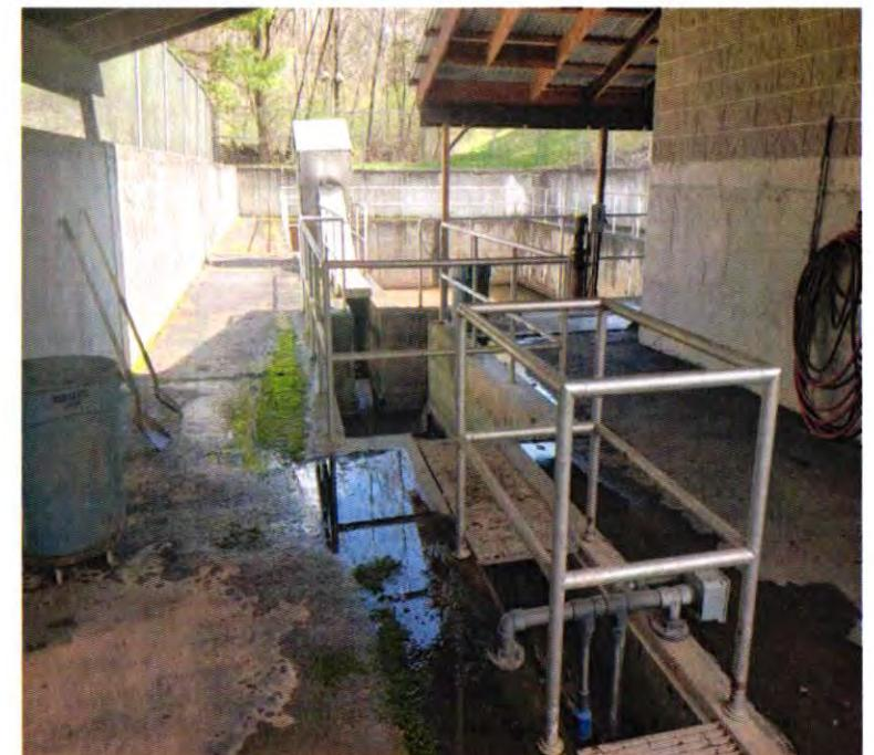
**NOTES:** Includes: bar screen, parshall flume, grit removal system, and controls.
