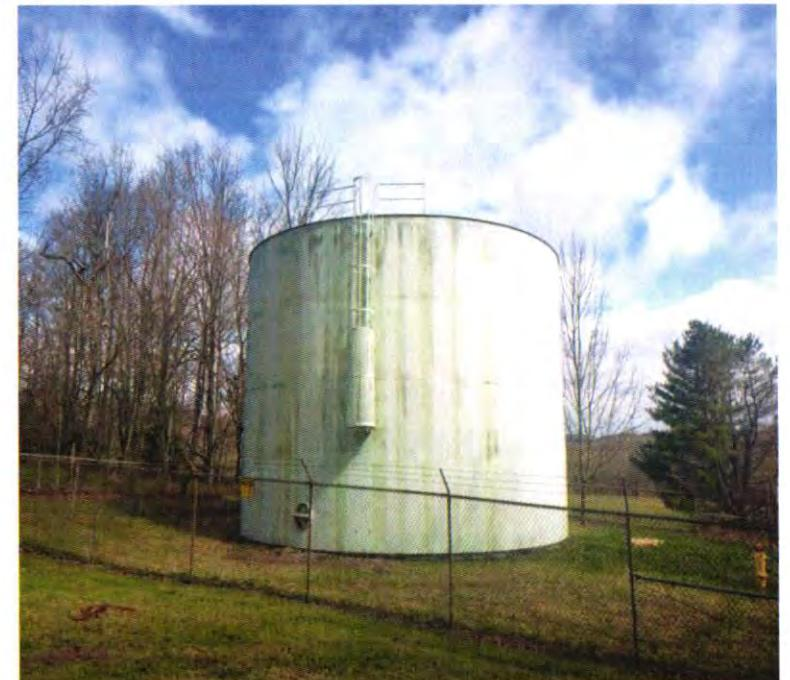
NOTES: 300,000 gallon capacity; welded steel tank. Site improvements include: fencing.
