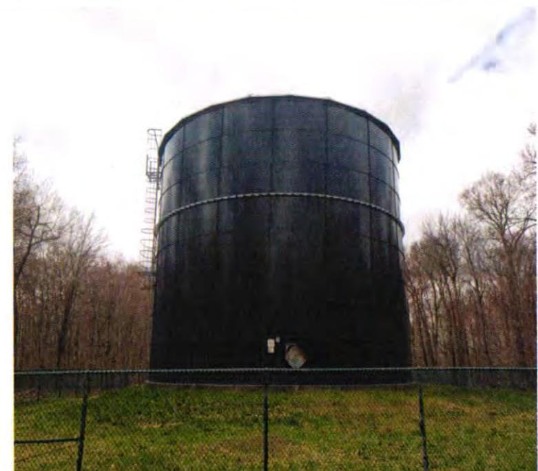
NOTES: 559,000 gallon capacity; bolted steel tank.
