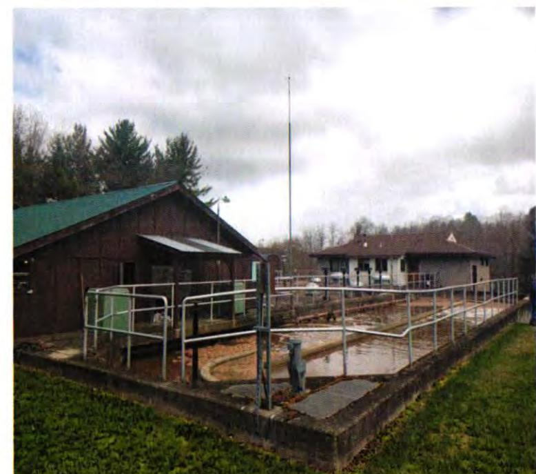
**NOTES:** .48mgd gallon capacity; includes: office, laboratory, garage, crane, 85k gallon sludge storage tank with 10hp pumps, (2) floating aerators, (3) 15hp recirculating pumps, (4) 5hp sludge pumps, (4) 15hp and (2) 5hp compressors, (2) uv systems, 230kw standby generator, valves, piping, and controls. Site improvements include: shed, fencing, and lighting.
