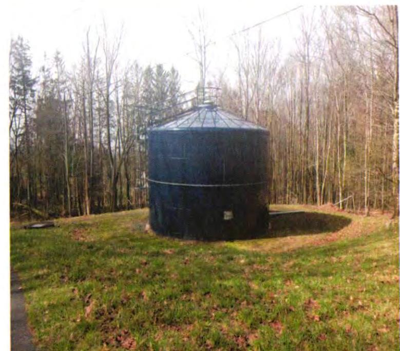
NOTES: 104,000 gallon capacity; bolted steel tank.
