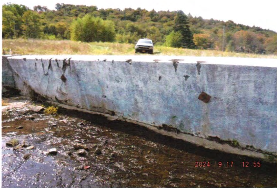
Photo 11 Dam ID# 162-4481 Tanzman Lake Dam 09/17/2024 Left downstream spillway side wall View looking left Note: lean of wall (out of plumb)
