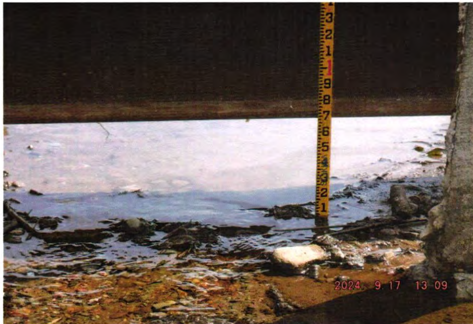
Photo 26 Dam ID# 162-4481 Tanzman Lake Dam 09/17/2024 Clearance below steel beam across spillway where concrete weir was located previously (apparently washed away or removed) Steel placed in support of sidewalls (?)
