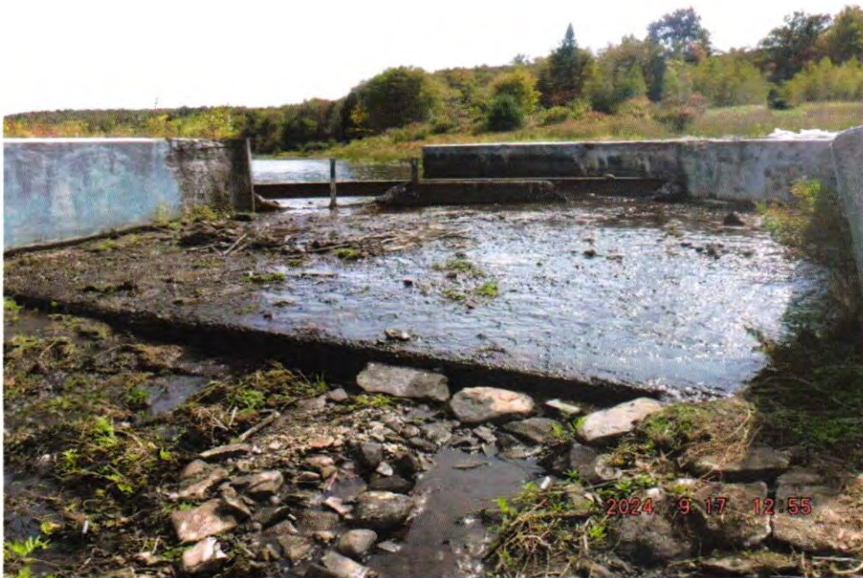
Photo 10 Dam ID# 162-4481 Tanzman Lake Dam 09/17/2024 Remnants of old concrete spillway weir and downstream apron View looking upstream
