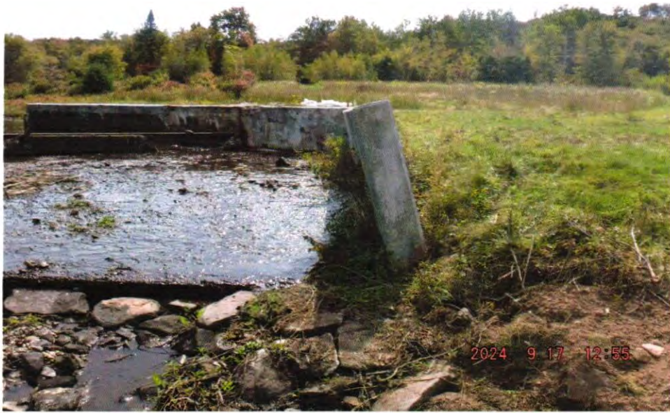
Photo 9 Dam ID# 162-4481 Tanzman Lake Dam 09/17/2024 Left downstream spillway side wall View looking upstream Note: lean of wall (out of plumb)
