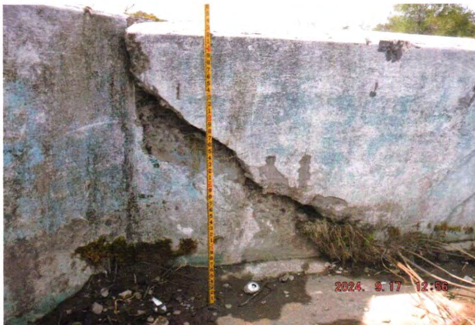
Photo 12 Dam ID# 162-4481 Tanzman Lake Dam 09/17/2024 Left downstream spillway side wall at joint View looking downstream Note: broken concrete and shift of wall
