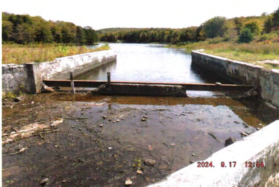
Photo 8 Dam ID# 162-4481 Tanzman Lake Dam 09/17/2024 Remnants of old concrete spillway weir View looking upstream
