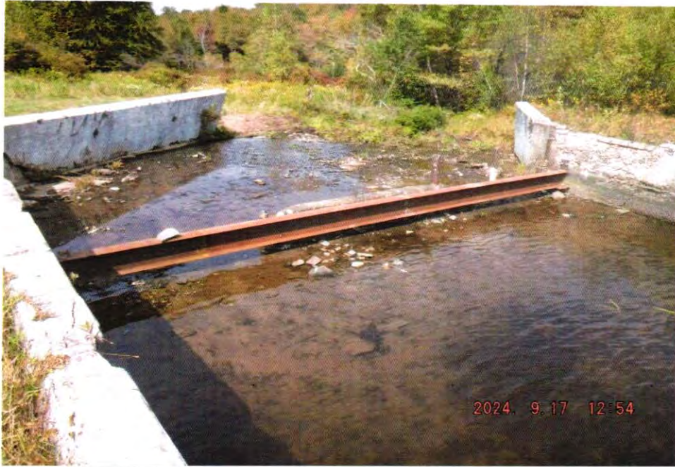
Photo 7 Dam ID# 162-4481 Tanzman Lake Dam 09/17/2024 Location of old concrete spillway weir (control section) View looking downstream
