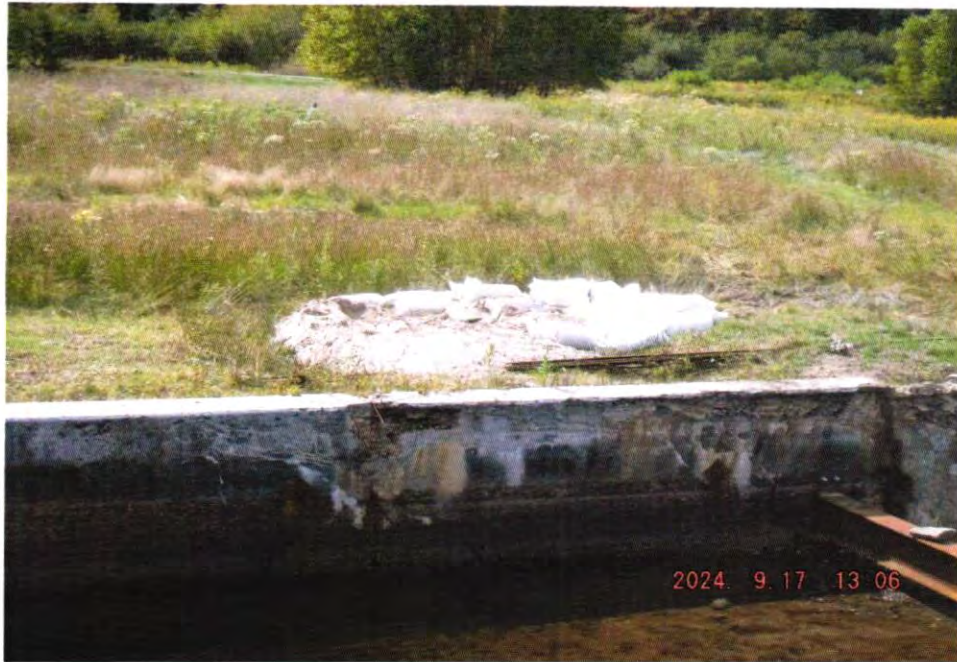
Photo 25 Dam ID# 162-4481 Tanzman Lake Dam 09/17/2024 Sand pile and sand bags behind left spillway sidewall
